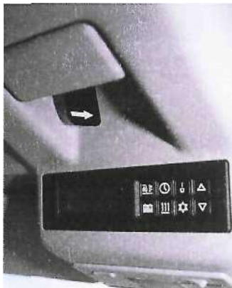
Roof console in the cab includes controls for heating and fridge.
